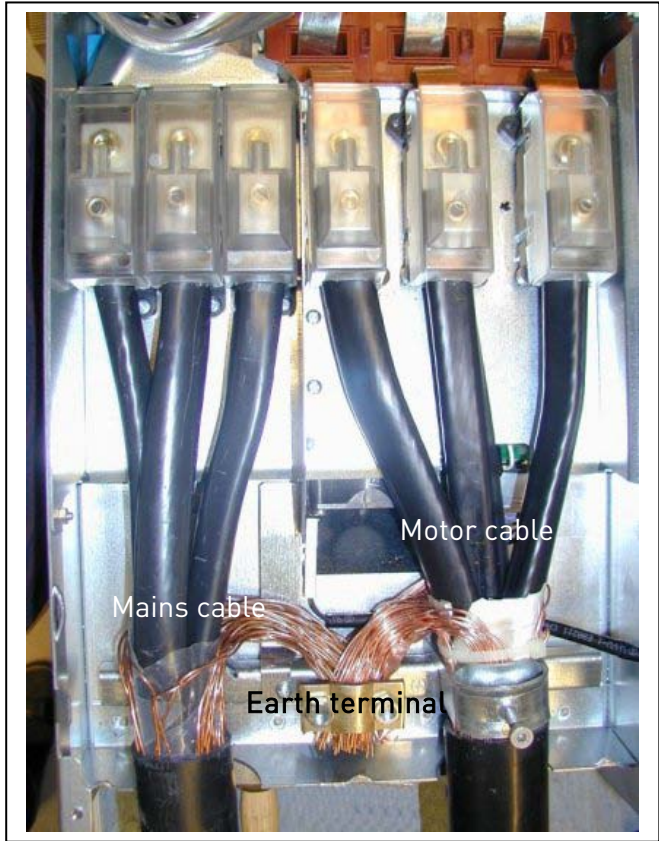
Figure 6-18. Cable installation in Vacon NXS/P, FR8
